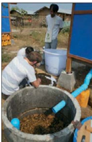
Tiger Toilet being installed (source: Bear Valley Ventures Ltd)
