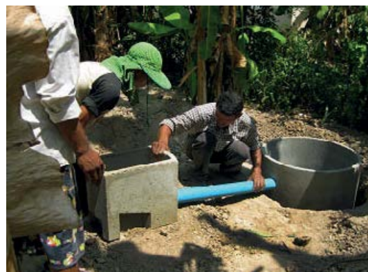
Installation of an iDE 'Easy Latrine'. Source : iDE Cambodia
