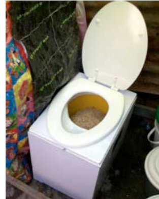
SOIL urine-diversion toilet. Source: Hystra
