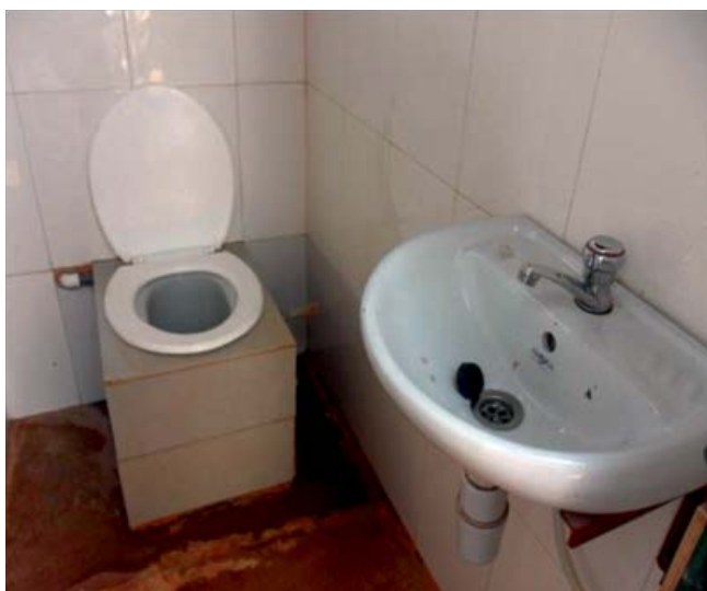
Biofil Microflush Toilet (source: www.biofilcom.org )
